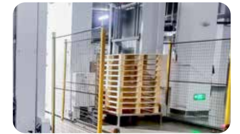
Automatic pallets feeding
